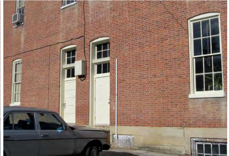
Painting of the First Floor Windows and Doors in South Wall Completed
