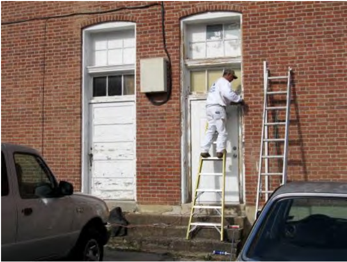
Painters preparing Surfaces of First Floor Doors and Transoms in South Wall for Painting
