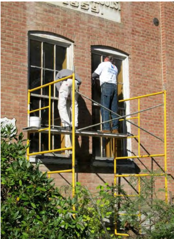
Painters preparing Surfaces of Windows and Window Frames in East Wall for Painting
